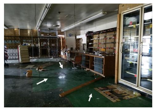
Photograph 5: View of the asbestos-containing 1' x 1' green floor tile over 9" x 9" dark green floor tile and mastic.
