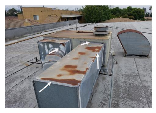
Photograph 3: View of the asbestos-containing duct sealant.
