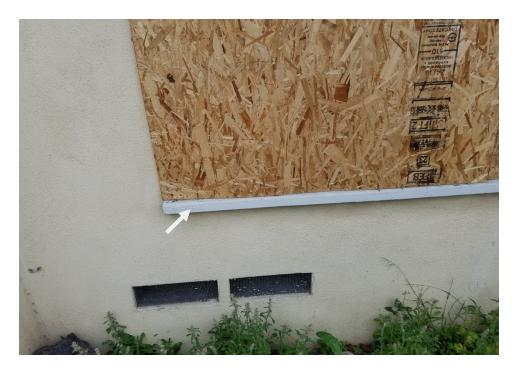
Photograph 12: View of the lead-containing white wood window frame.
