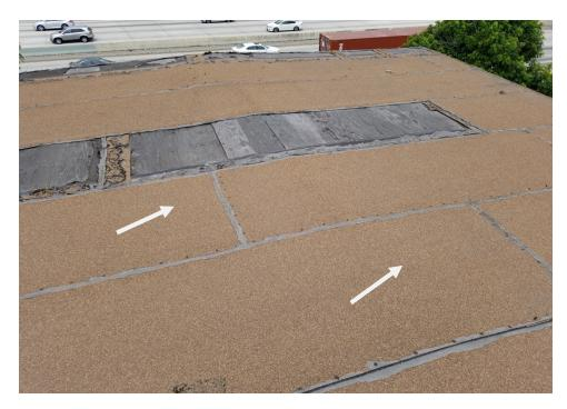
Photograph 16: View of the asbestos-containing rolled roofing.
