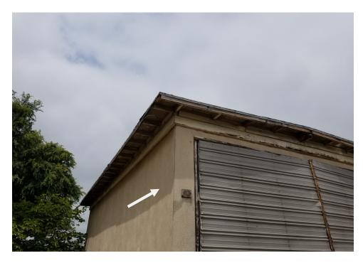
Photograph 17: View of the asbestos-containing stucco.
