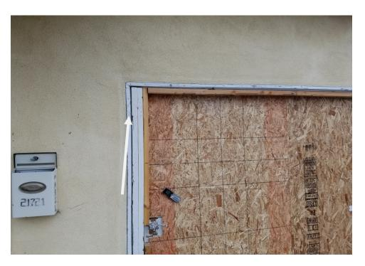
Photograph 13: View of the lead-containing white wood garage door frame.
