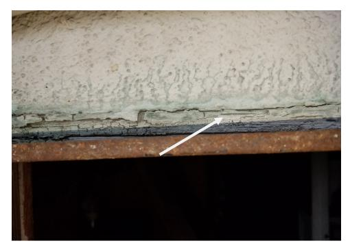
Photograph 6: View of lead-containing beige wood door frame.
