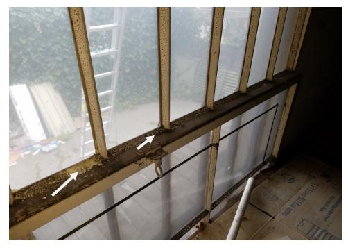
Photograph 4: View of the asbestos-containing window putty.
