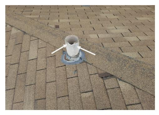
Photograph 9: View of asbestos-containing transite pipe.
