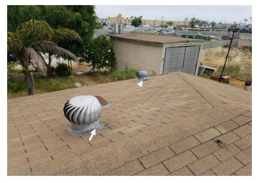
Photograph 10: View of the asbestos-containing roof mastic.
