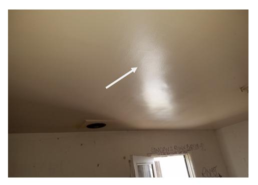
Photograph 14: View of the lead-containing white plaster ceiling.
