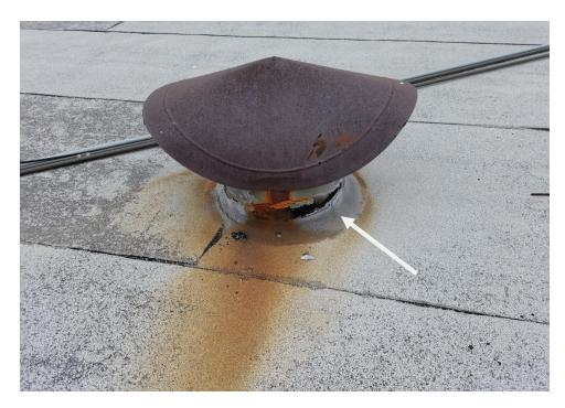
Photograph 2: View of the asbestos-containing roof mastic.
