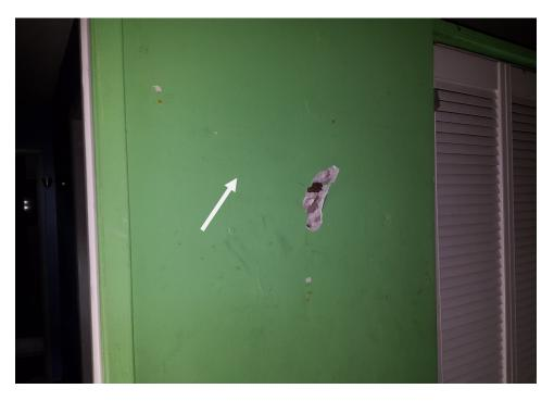
Photograph 11: View of the asbestos-containing button board with plaster.
