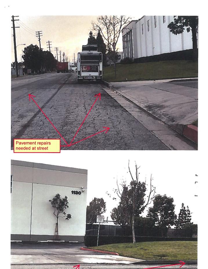
curb and gutter repairs (low spot constant ponding)
