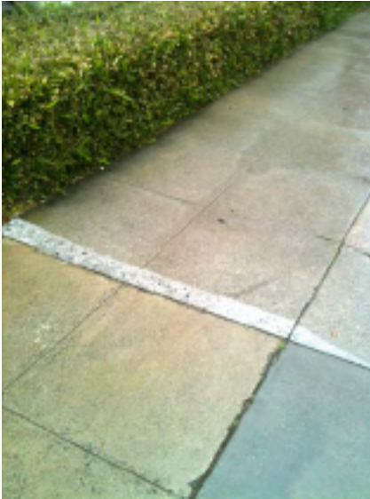
1/2 to 1 inch high Repair by Precision Saw Cutting
