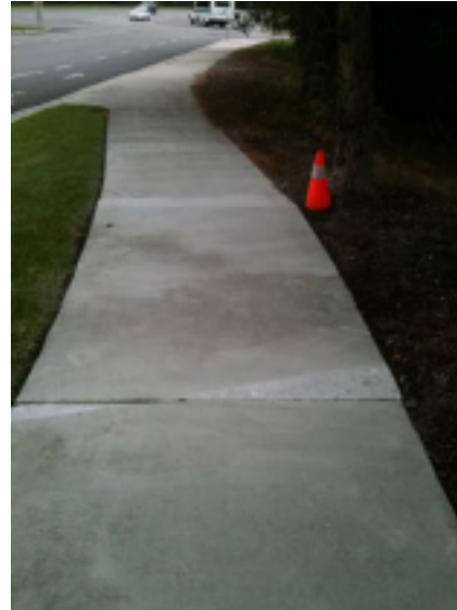
1 to 1 1/2 Inches High Repair by Precision Saw Cutting
