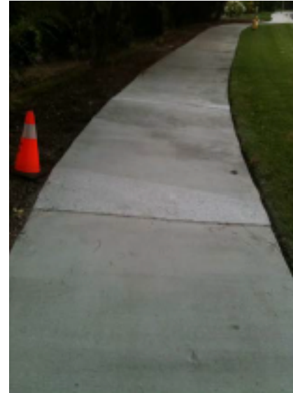
1 1/2 to 2 Inches High Repair by Precision Saw Cutting
