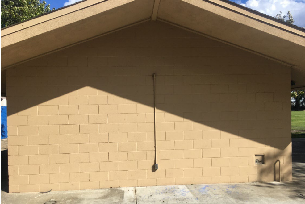
West Exterior Wall – Snack Bar
