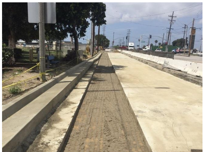
New Curb & Gutter and Base along 223 rd Street across from Del Taco
