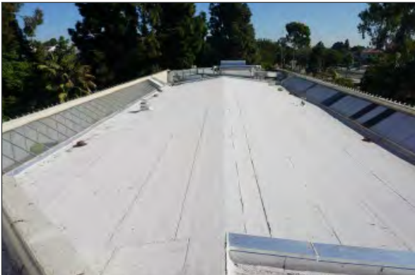
View of the roof and skylights on the east wing (WJE, 2023).
