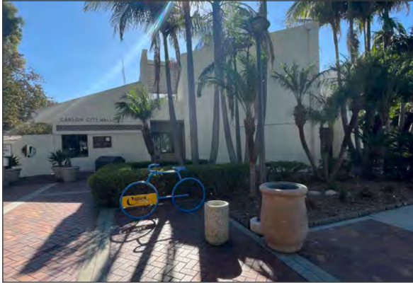
View south of the north wing's north façade (ARG, 2023).
