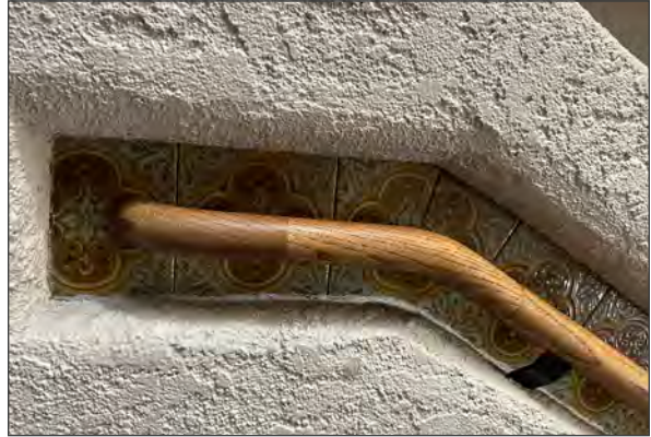
Detail of polychromatic tile at central staircase (ARG, 2023).
