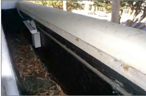
Typical exterior second floor planter (WJE, 2023).
