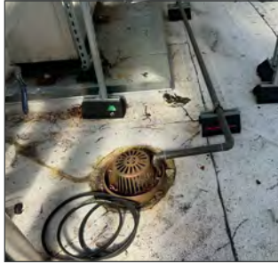
Roof scuppers (ARG, 2023).
