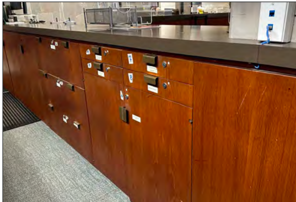
Hardwood public service counter with laminated top and brass pulls in the east wing, first floor (ARG, 2023).
