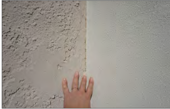
Original textured stucco (left) and new smooth stucco (right) (WJE, 2023).
