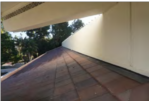
Tile roof on the lower volume of the east wing (WJE, 2023).
