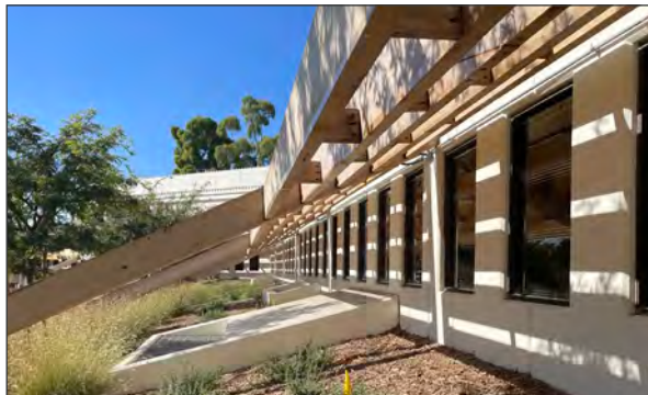
Punched aluminum-framed windows (ARG, 2023).
