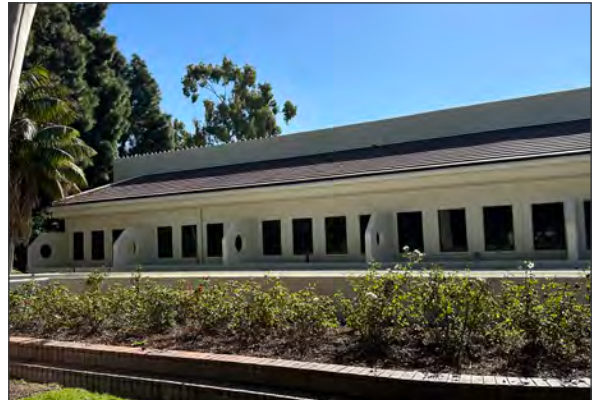
View southeast of the east wing’s north façade (ARG, 2023).
