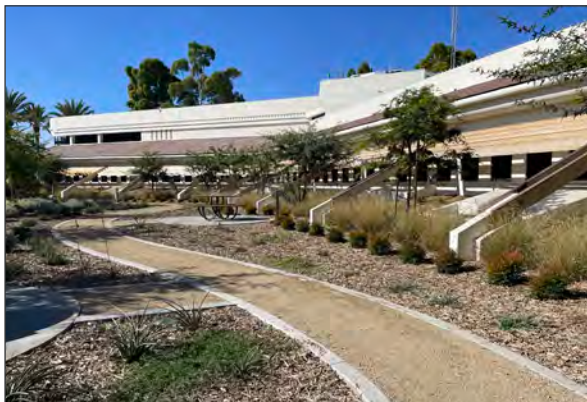
View west of the east wing’s south façade (ARG, 2023).
