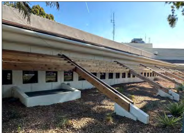
Fixed bronze aluminum windows fronted by a wood trellis at the north wing, west façade (ARG, 2023).
