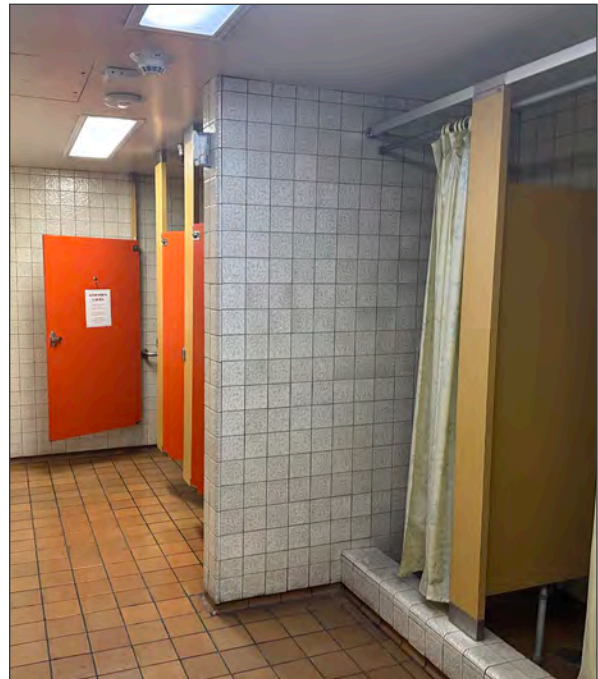
Basement women’s restroom (ARG, 2023).
