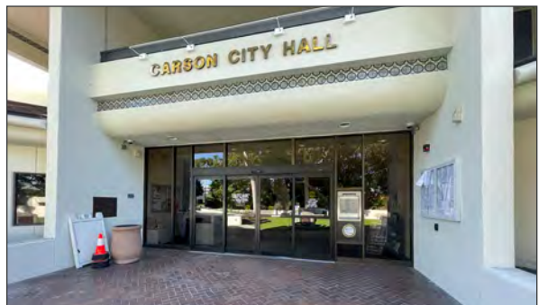
Recessed entry, fixed tinted glazing, and metal depository box at the southwest wing, north façade (ARG, 2023).
