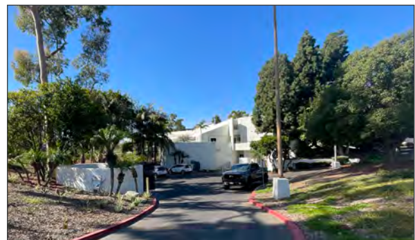
View west of the east parking/loading area (ARG, 2023).
