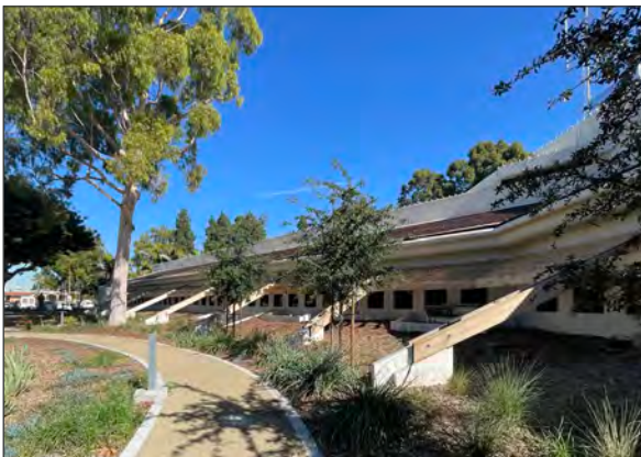
View northeast of the north wing's west façade (ARG, 2023).
