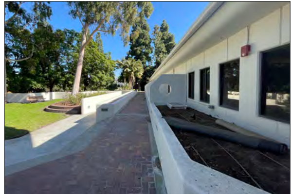
Fixed bronze aluminum windows divided by concrete fins at the east wing, north façade (ARG, 2023).
