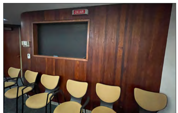
Wood plank wall finishes in the council chambers (ARG, 2023).
