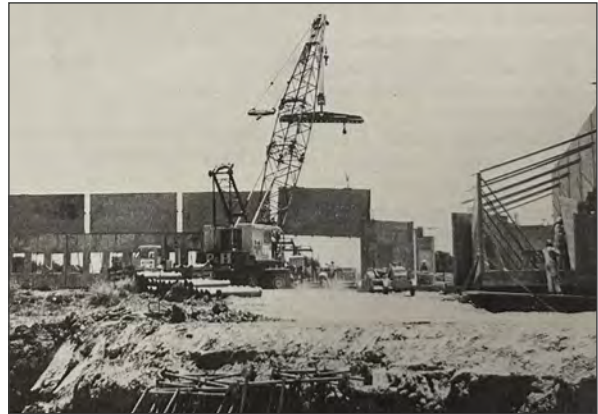
City Hall under construction, 1974 (Trejos, My Carson Your Carson ).
