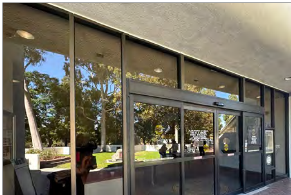
Aluminum-framed storefronts at north entrance (ARG, 2023).
