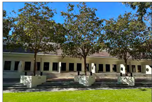
View west of the north wing's east façade (ARG, 2023).
