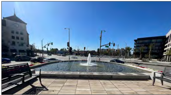
South entrance plaza circular fountain (ARG, 2023).
