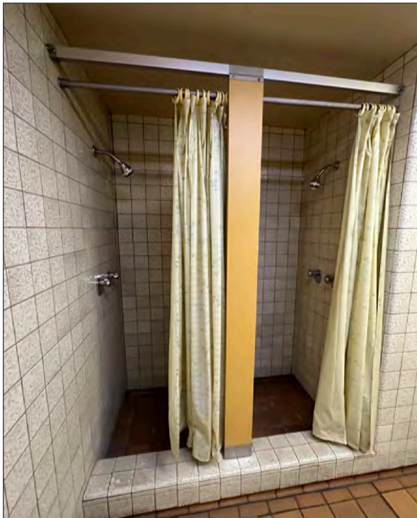
Basement restroom with plaster ceiling, ceramic tile walls, quarry tile flooring, and showers (ARG, 2023).
