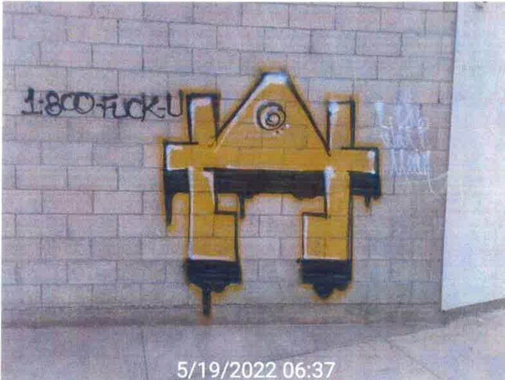
TG22-0087036 05/19/22 Western Ave and Plaza del Amo
