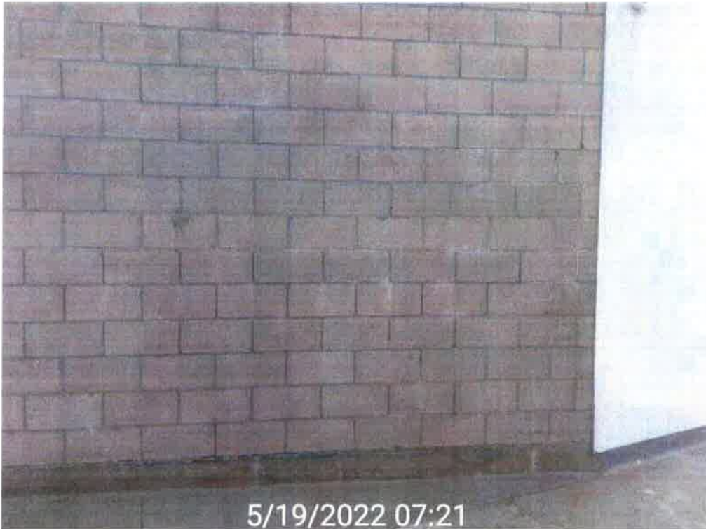
TG22-0087036 05/19/22 Western Ave and Plaza del Amo
