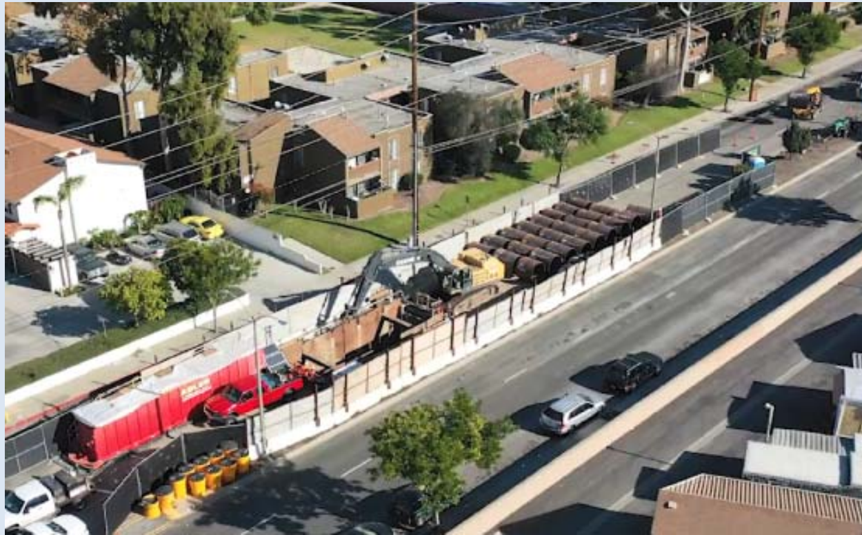
Second Lower Feeder Access Site Photo courtesy of Black & Veatch, 78" steel water pipe
