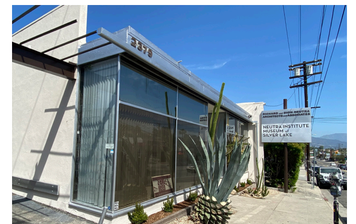
View northeast of the office building
